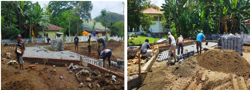
Gambar 4.7 Proses Pemasangan Grass Block
