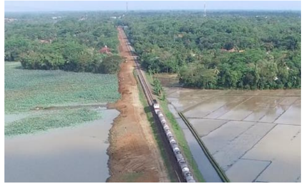
Figure 1. Existing railway track condition
