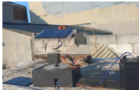
Figure 12. Testing the tracking solar panel
