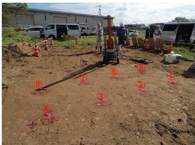
Photo 1. Surface condition of the survey site.
