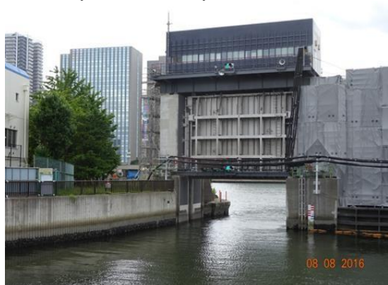
Figure 2. A flood gate under the aseismic reinforcing work
