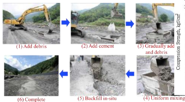
Figure 5 The process of In-situ Mixing Method (Premix)
