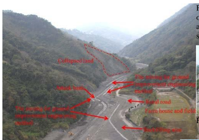
Figure 4 The mixing land improvement engineering method improvement structure, showing the objects to be protected
