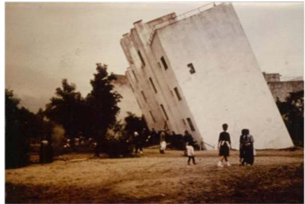
Figure 3. Damage to a RC four story building due to liquefaction (1964 Niigata earthquake, Japan)
