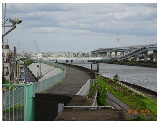
Figure 1. Below-sea-level Area of Tokyo (BAT)
