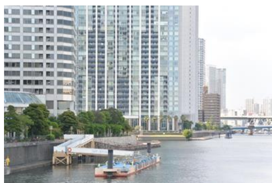
Figure 4. Seawall at Tenozu
