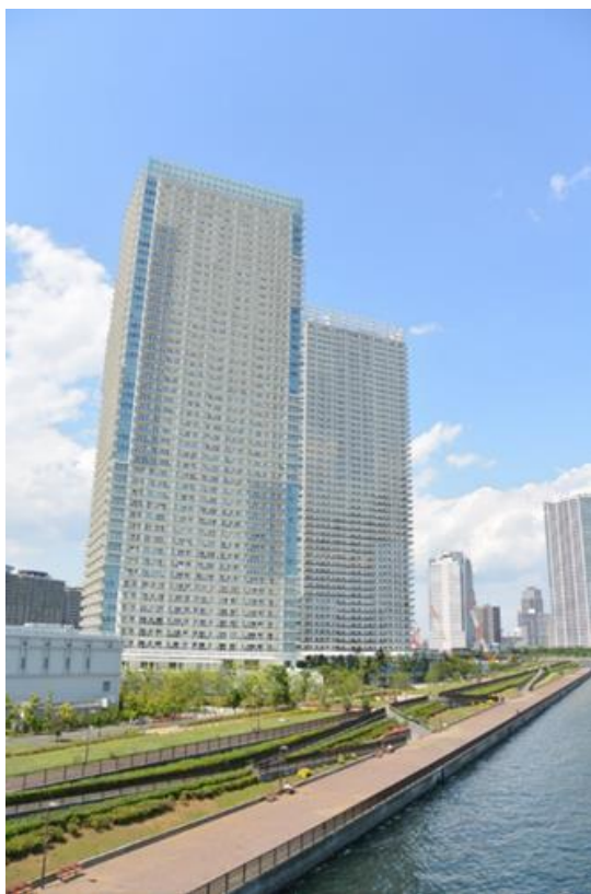
Figure 6. Seawalls at Kachidoki
