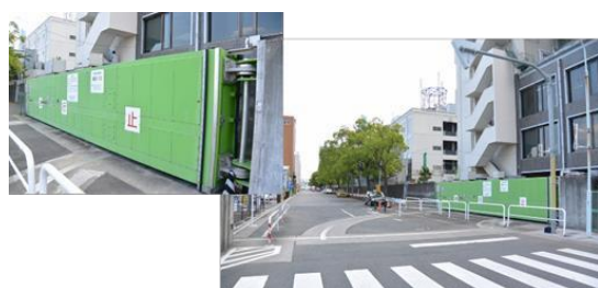
Figure 3. Floodwall gate at Harumi
