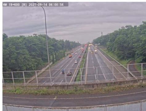
Figure 4. Research location, Jagorawi Toll Road KM 19+600
