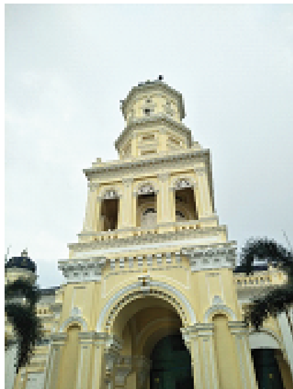
Figure 1: One of Sultan Abu Bakar Mosque Minarates.
