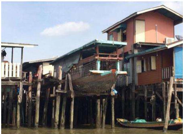
Picture 02-03 Stilt housing and boat house lifted on the wooden beam
