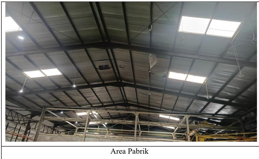
*Gambar 4. 6 Pencahayaan Alami Gedung PT. Voestalpine Bohler Welding Asia Pasific
