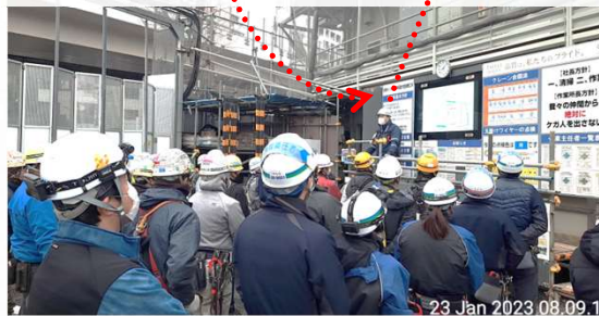
Site Manager (SM) memberikan arahan di setiap TBM
