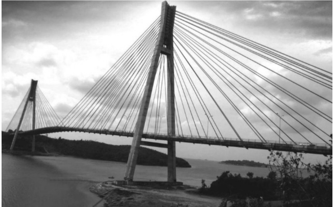
Gambar 1.7 Cable-Stayed Bridge
