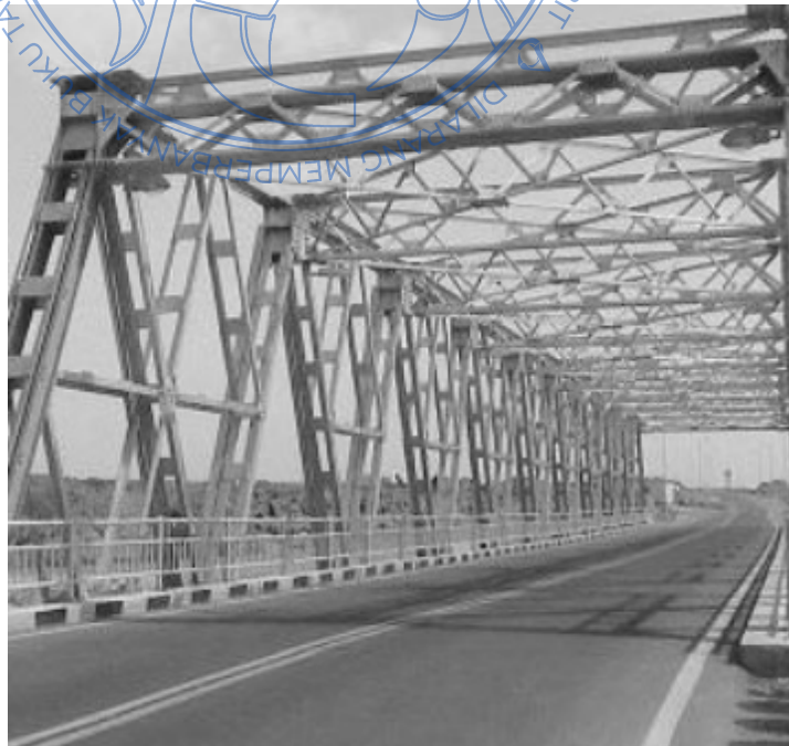
Gambar 1.3 Truss Bridge
