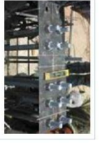
Setting up Anchor Bolt
