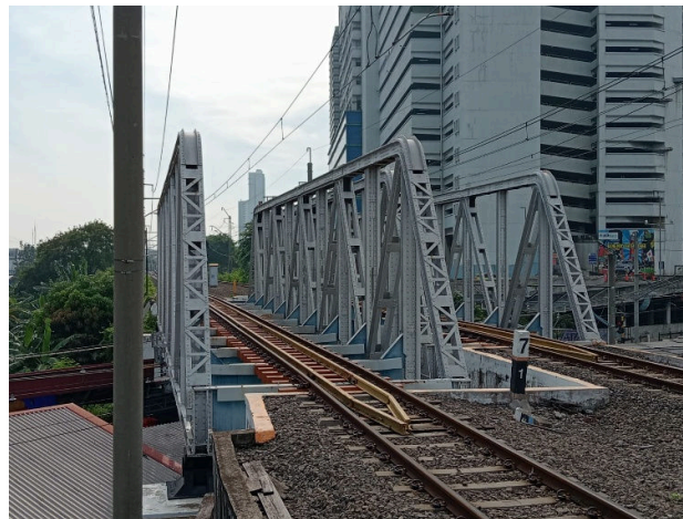
Figure 2. Railway bridge in Jakarta Source: Documentation, 2025
