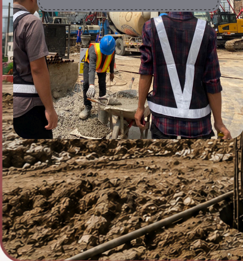
Slumb Test Beton
