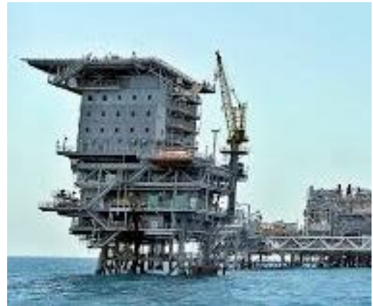
Gambar 3.3 Bangunan Living Quarters Anjungan Lepas Pantai PT.X.
