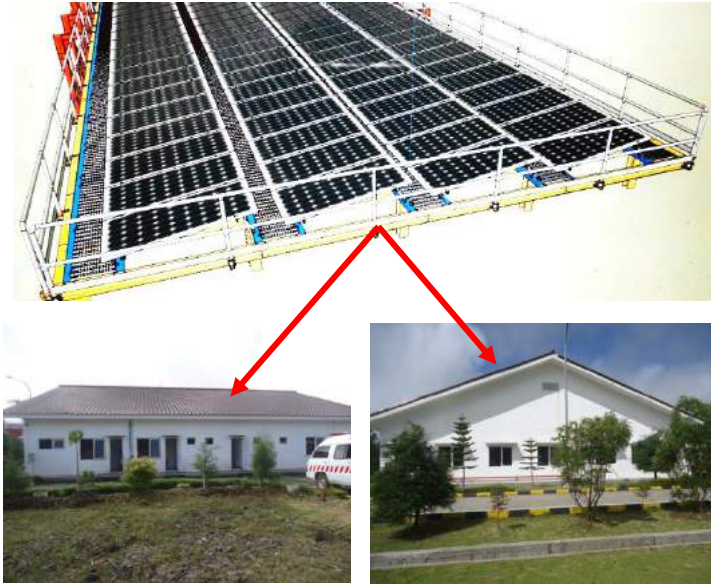
Gambar 6.16 Potensi Rooftop (atap) di Bangunan Gedung Admin
