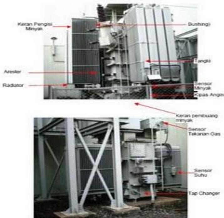
Gambar 4.3. Transformator Tipe Conventional Beradiator (Trafindo, 2005)
