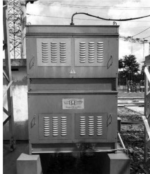
Gambar 1. Sistem Neutral Grounding Resistance (NGR) di Gardu Induk Cawang Lama
