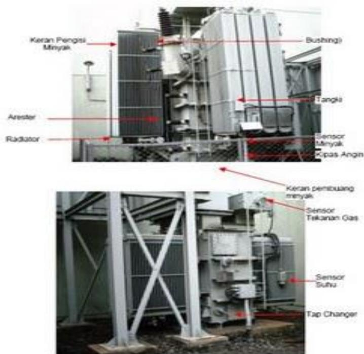
Gambar 2. Transformator Tipe Conventional Beradiator (Trafindo, 2005)
