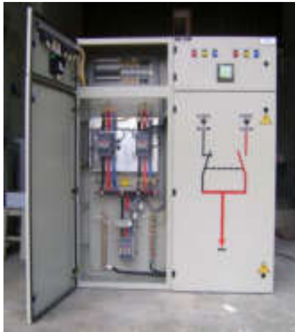
Panel Automatic Transfer Switch (ATS)
