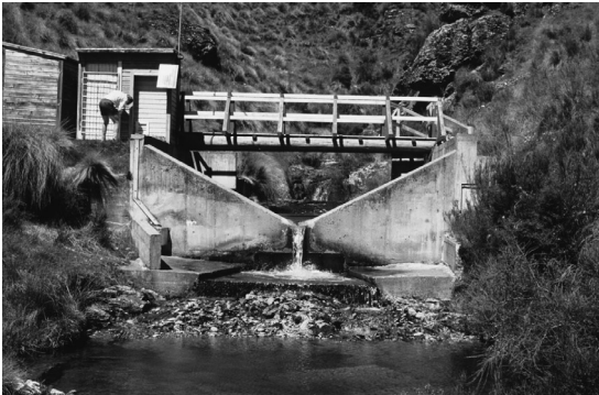
Figure 5.11 A V-notch weir. The water level in the pond behind the weir is recorded continuously.
