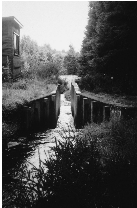
Figure 5.12 A trapezoidal flume. The stream passes through the flume and the water level at the base of the flume is recorded continuously.
