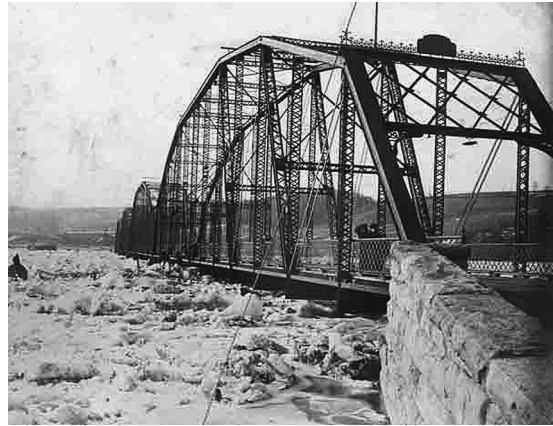
Figure 4.14 Susquehanna river ice jam and flood which destroyed the Catawissa Bridge in Pennsylvania, USA on 9 March 1904.
