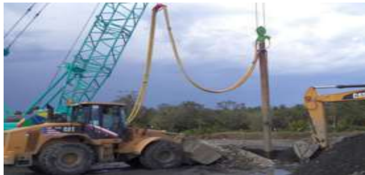
Gambar 1. 4 Stone Column Soil Improvement _(Menard, 2016)
