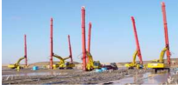
Gambar 1. 2 PVD Preloading Soil Improvement _(Menard, 2016)
