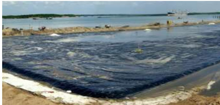
Gambar 1. 3 PVD Preloading Vacuum Soil Improvement _(Menard, 2016)
