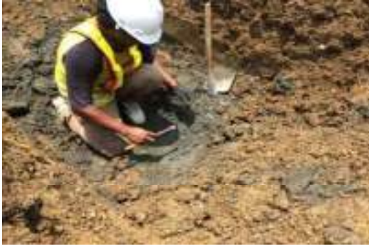
Test Pit No.2
