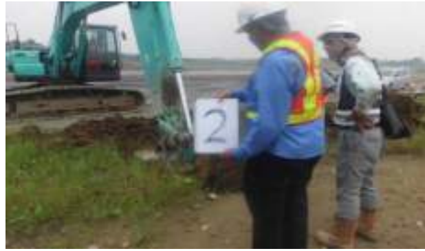
Test Pit Location-2
