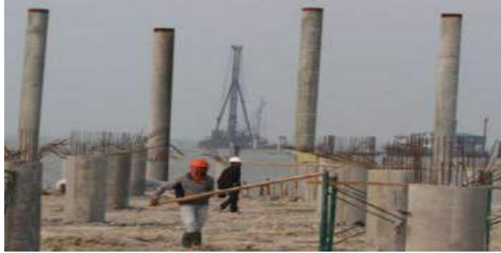
Gambar 1. 6 Tiang Pancang Soil Improvement (Menard, 2016)
