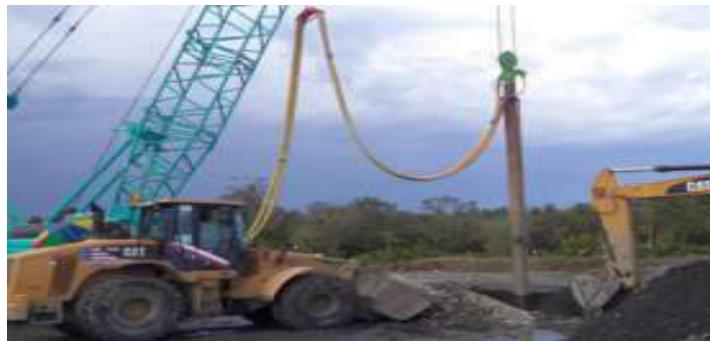
Gambar 1. 4 Stone Column Soil Improvement _(Menard, 2016)
