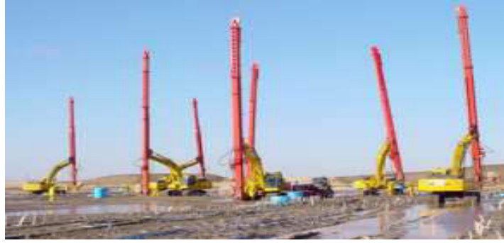
Gambar 1. 2 PVD Preloading Soil Improvement _(Menard, 2016)
