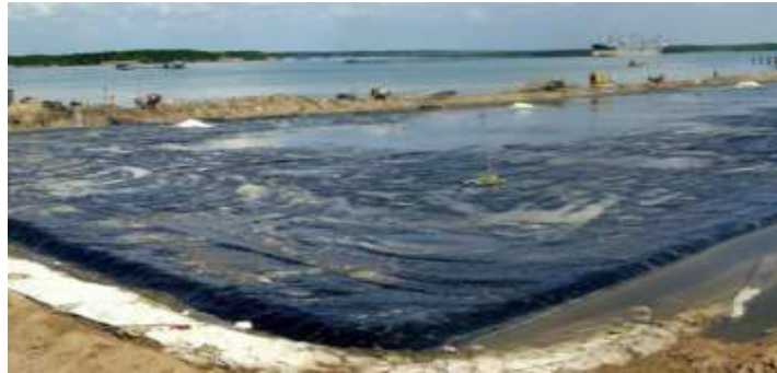
Gambar 1. 3 PVD Preloading Vacuum Soil Improvement _(Menard, 2016)
